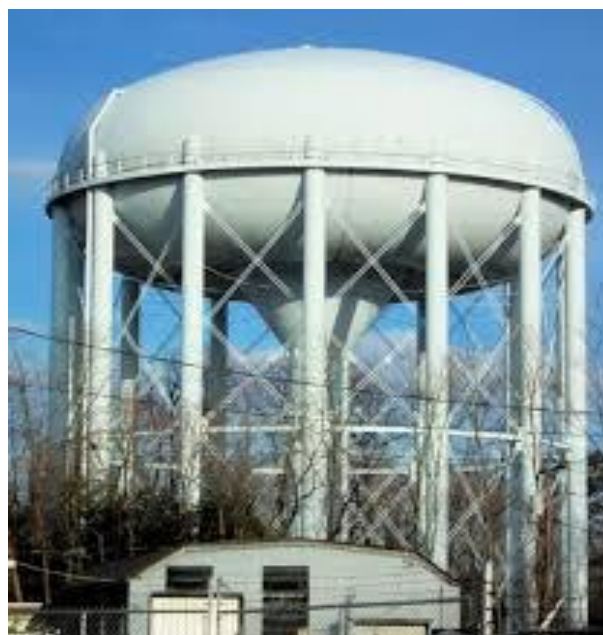
Fig. 1.4: Elevated Service Reservoir
