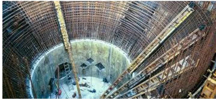
Fig .1.2: Raw Water Reservoir
